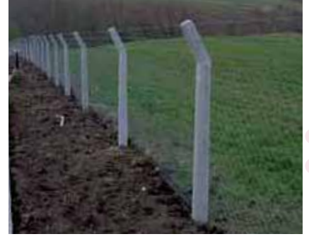
Beton direkli örgü tel uygulamaları. (Direk her 3 metrede 1 adet. Payanda onbeş direkte 1 çift.) Chain link fence application with concrete posts. (Post Usage: 1 pc/every 3 m, Brace Usage: 1 pair / every 15 post)
