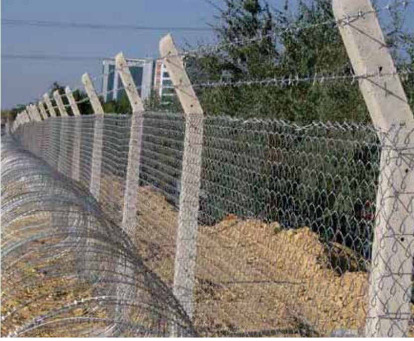
Beton direkli örgü tel uygulamaları. (Direk her 3 metrede 1 adet. Payanda onbeş direkte 1 çift.) Chain link fence application with concrete posts. (Post Usage: 1 pc/every 3 m, Brace Usage: 1 pair / every 15 post)
